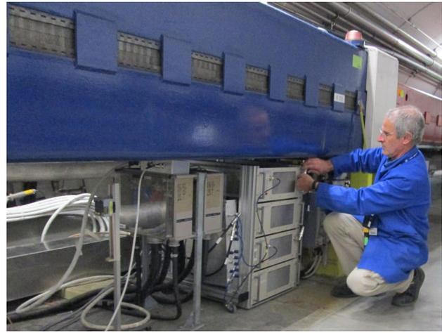
Figure 15: Two wideband 5 - 1000 MHz amplifiers installed in the SPS tunnel as part of the upgrade to use 1 GHz bandwidth vertical kicker striplines. Two more additional amplifiers will be installed in 2016 to power the second stripline.
